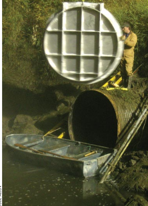
The new tide gate during installation.
